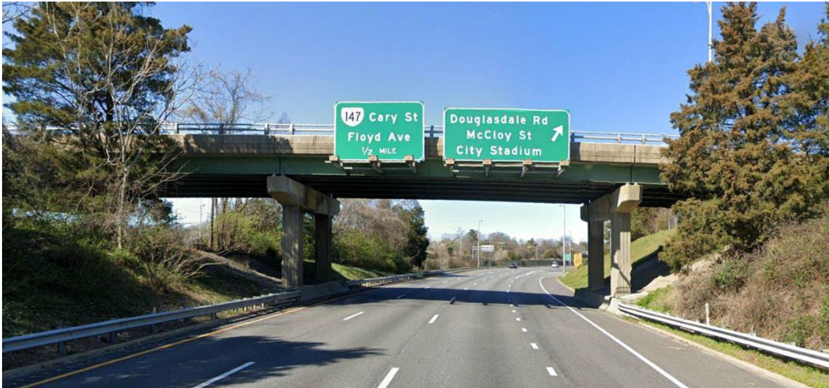
Douglasdale road over NB Powhite Pkwy VA-76 and CSX Railroad
