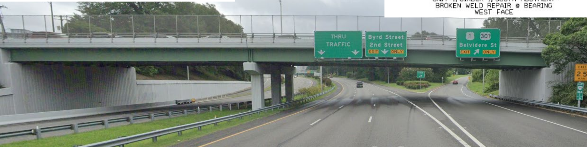
Bridge 48, S. Harrison Street over Downtown Expressway East Bound Direction Shown
