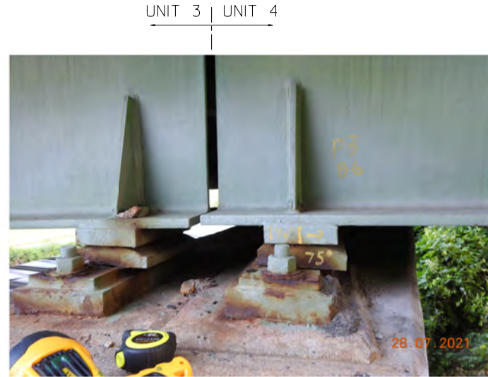
BRIDGE 13, PIER 3 UNIT 3, STRINGER 1-6 UNIT 4, STRINGER 5-6 BEARING MISALIGNED
