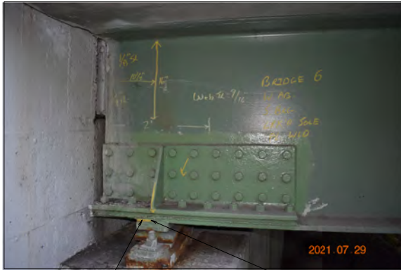
UNIT 1, BEAM 10, WEST ABUTMENT BROKEN WELD REPAIR @ BEARING SOUTH FACE
