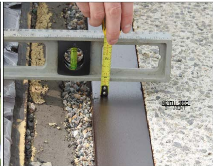
TYPICAL UNLEVEL DECK JOINT
