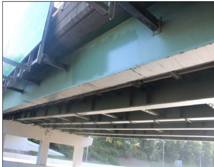
BRIDGE 47 SPAN 1, STRINGER 1 REPAIR 2
