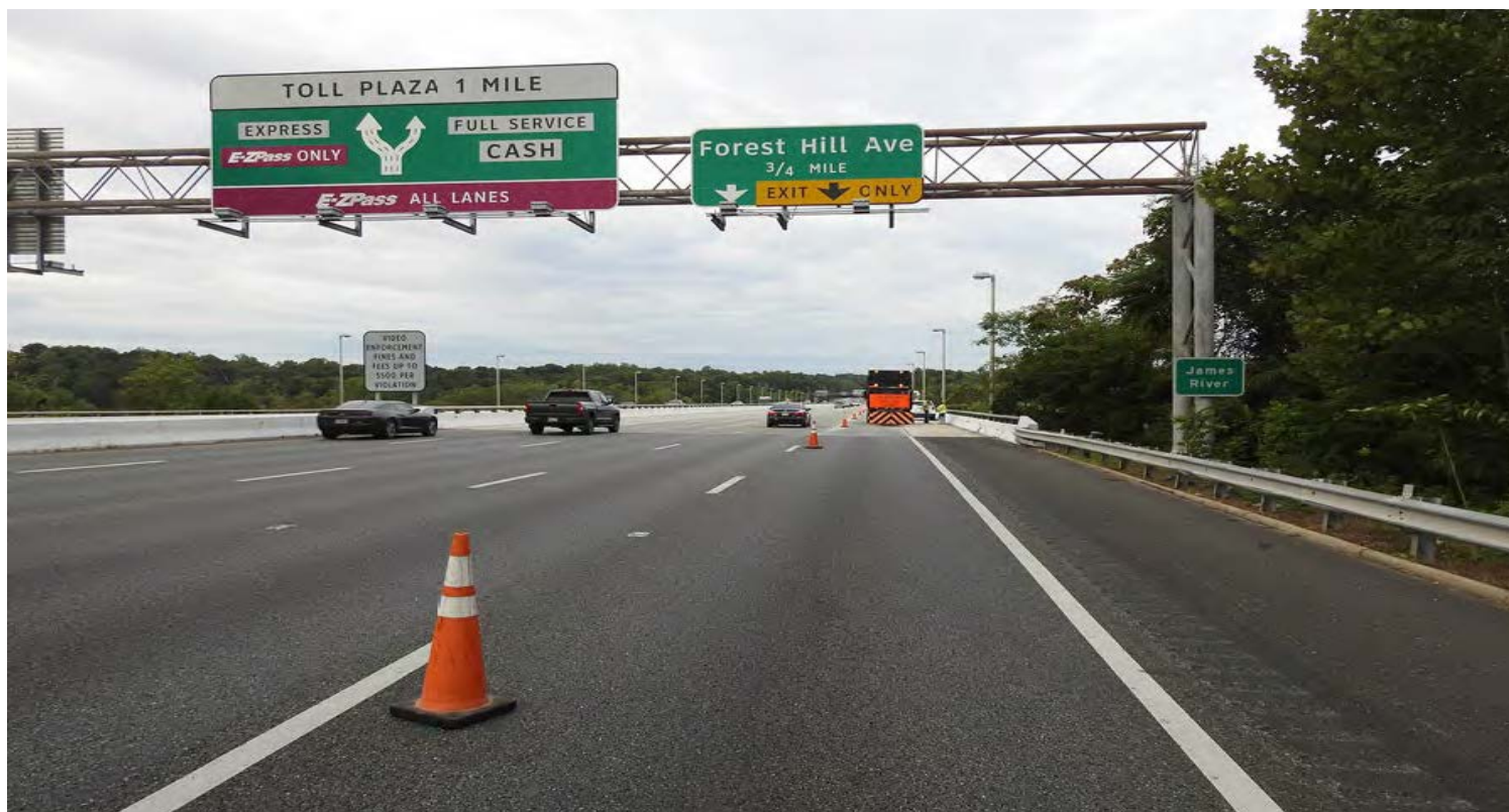
SB Powhite Parkway Over James River Kanawha Canal and CSX
