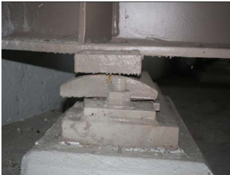
BRIDGE 62, WEST ABUTMENT TYPICAL GIRDERS 1-4 CLOSE-UP VIEW
