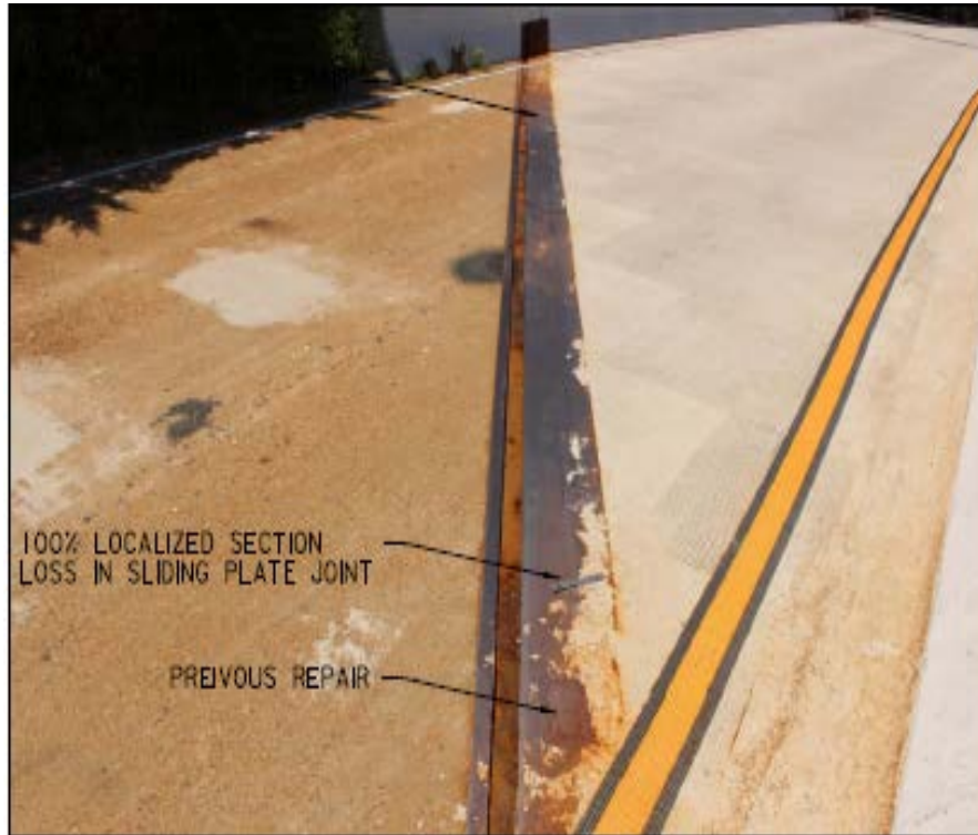
BRIDGE 17, NORTH ABUTMENT S. FLOYD AVE.
