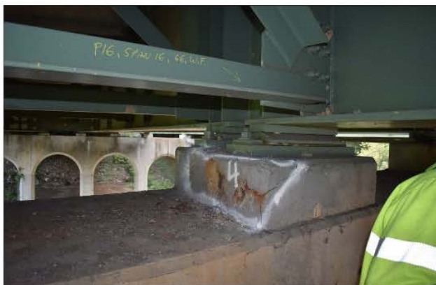
TYPICAL ORIGINAL BEARINGS
