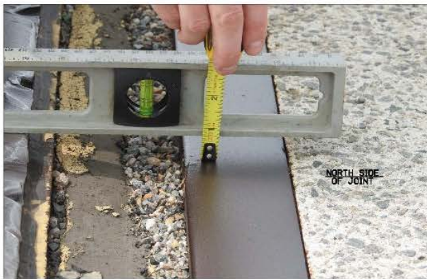
TYPICAL UNLEVEL DECK JOINT
