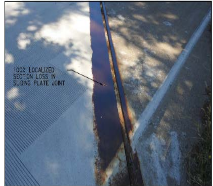
BRIDGE 17, NORTH ABUTMENT S. CARY ST.
