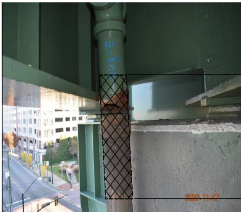
EXISTING DRAIN PIPE @ UNIT 2, PIER 1
