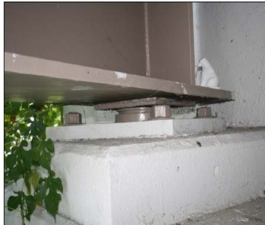
BRIDGE 62, WEST ABUTMENT GIRDER 5 BEARING FOR INFORMATION ONLY
