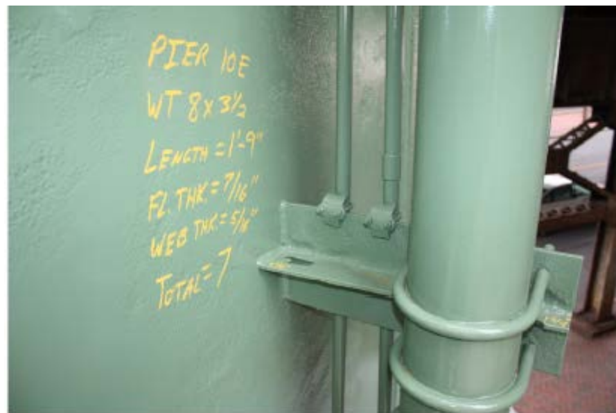
BRIDGE 67, PIER 10E CLOSE-UP VIEW
