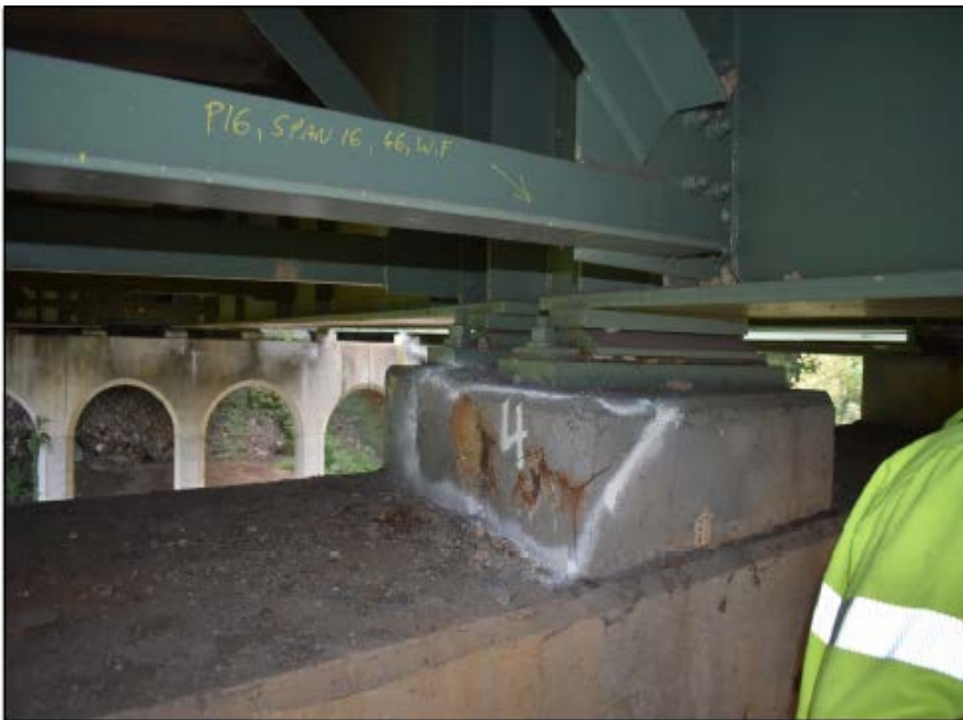
TYPICAL ORIGINAL BEARINGS
