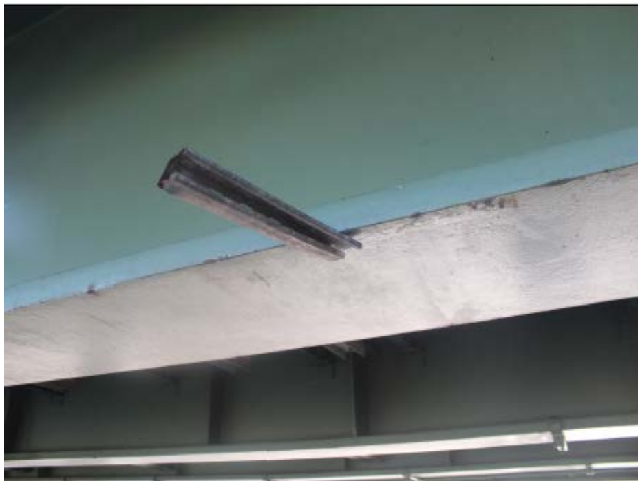
BRIDGE 47 SPAN 1, STRINGER 1 REPAIR 1
