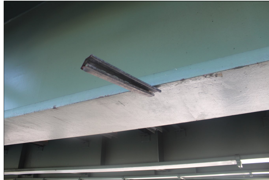
BRIDGE 47 SPAN 1, STRINGER 1 REPAIR 1
