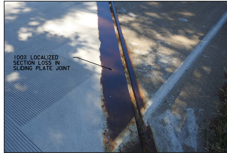
BRIDGE 17, NORTH ABUTMENT S. CARY ST.
