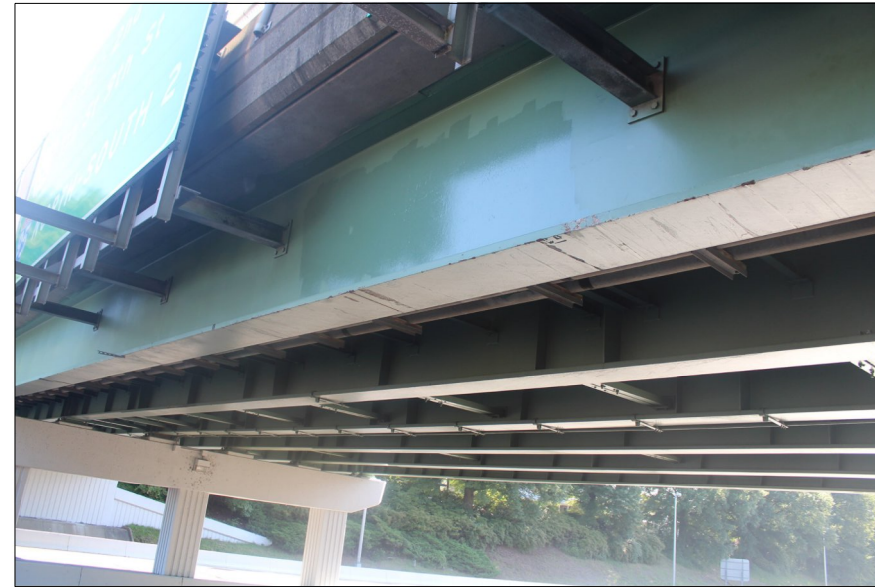
BRIDGE 47 SPAN 1, STRINGER 1 REPAIR 2
