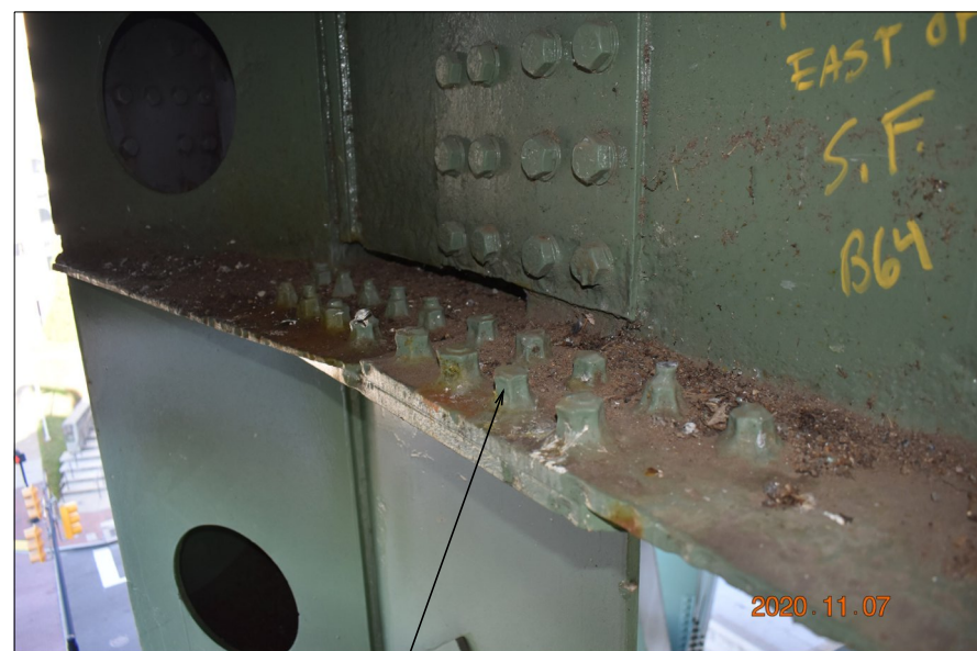
REPLACE 18 - 7/8" DIA. BOLTS WITH NEW BOLTS
