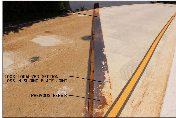
BRIDGE 17, NORTH ABUTMENT S. FLOYD AVE.
