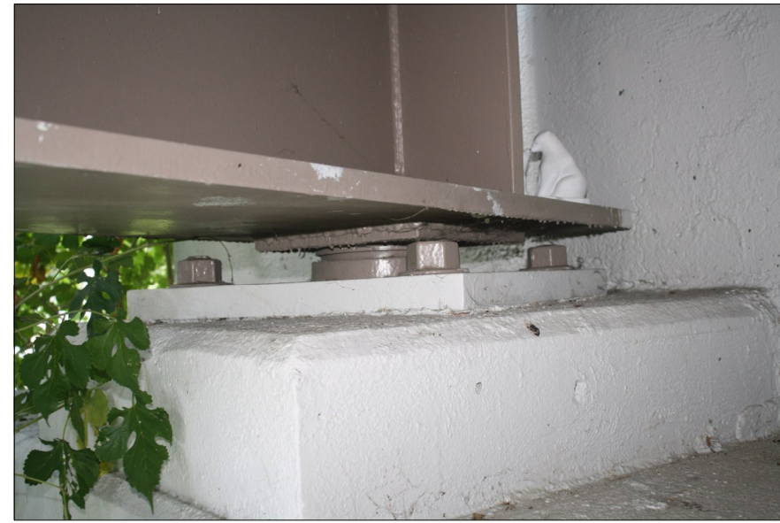
BRIDGE 62, WEST ABUTMENT GIRDER 5 BEARING FOR INFORMATION ONLY
