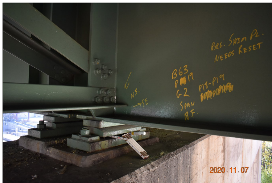
PIER 19, UNIT 20, GIRDER 2 EXISTING CONDITION
