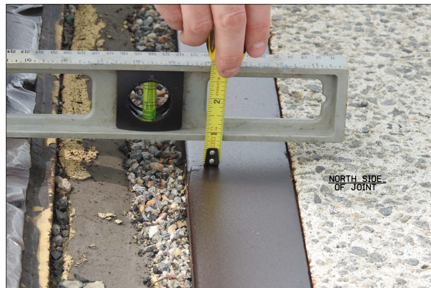
TYPICAL UNLEVEL DECK JOINT
