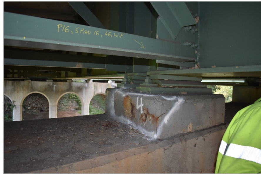
TYPICAL ORIGINAL BEARINGS
