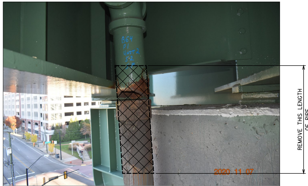
EXISTING DRAIN PIPE @ UNIT 2, PIER 1
