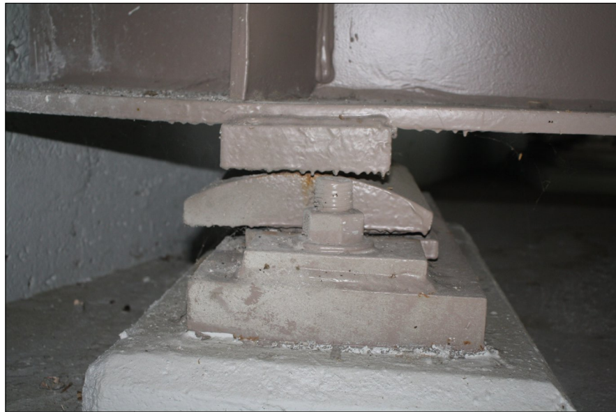
BRIDGE 62, WEST ABUTMENT TYPICAL GIRDERS 1-4 CLOSE-UP VIEW
