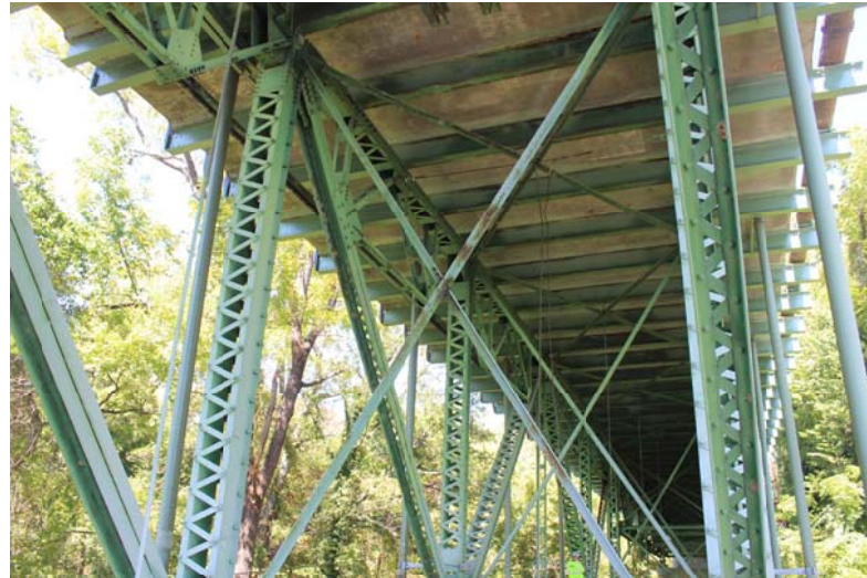
SPAN 13 SWAY FRAME
