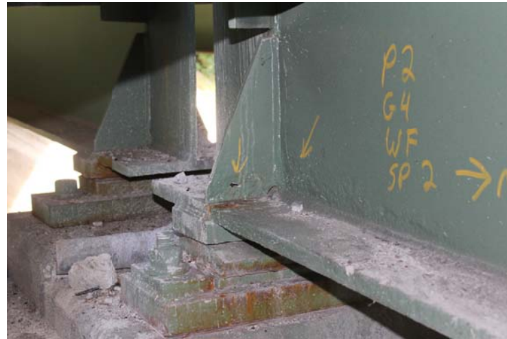
BRIDGE 11, PIER 2 BEAM 4
