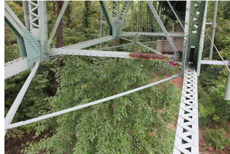
SPAN 13 LOWER STRUT
