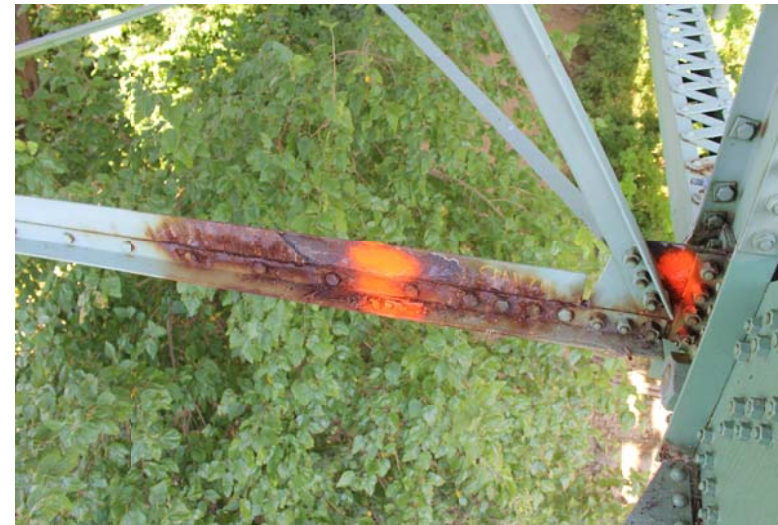
SPAN 13 LOWER STRUT CONNECTION PLATE
