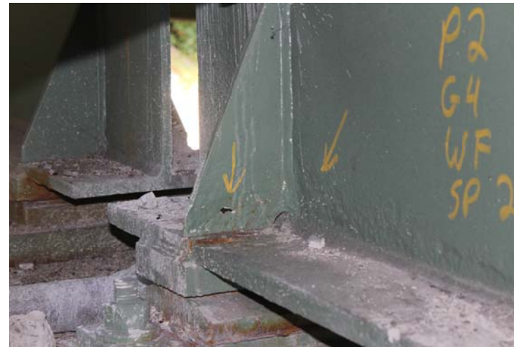
BRIDGE 11, PIER 2 BEAM 4, CLOSE-UP VIEW
