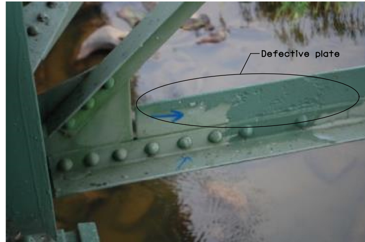
UNIT 11 LATERAL BRACING ANGLE IN WEST TRUSS
