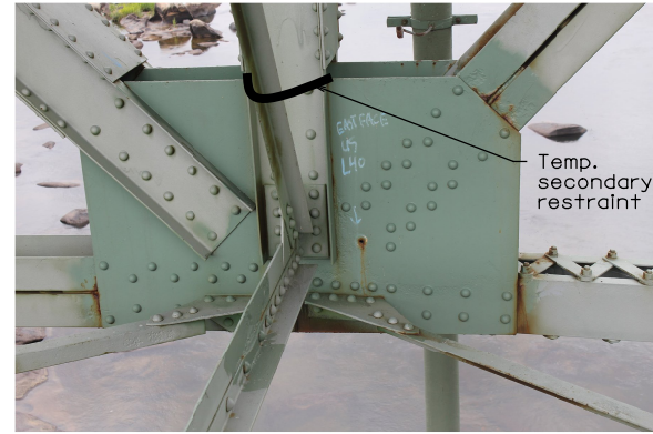
DETAIL D Temporary restraint/tie off
