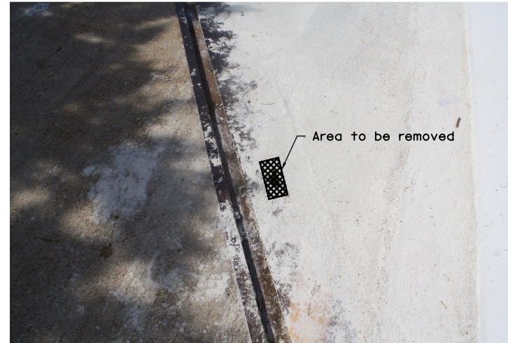
BRIDGE 17, NORTH ABUTMENT S-FLOYD
