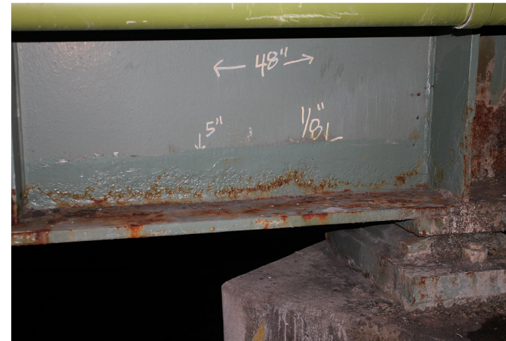
BRIDGE 5, PIER 5 STRINGER S41
