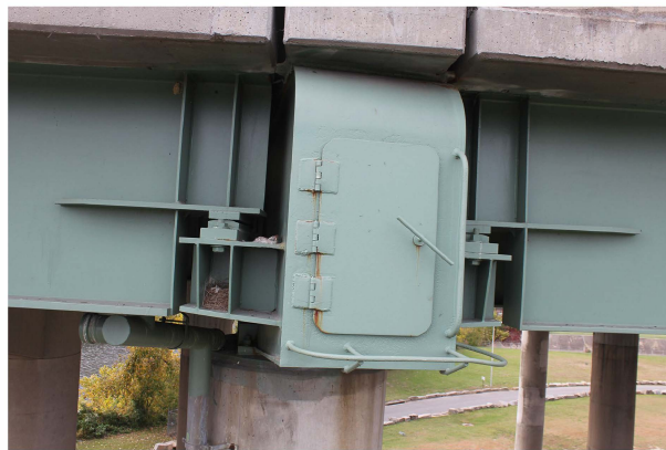
BRIDGE 65 PIER 6 - Hinge Repair
