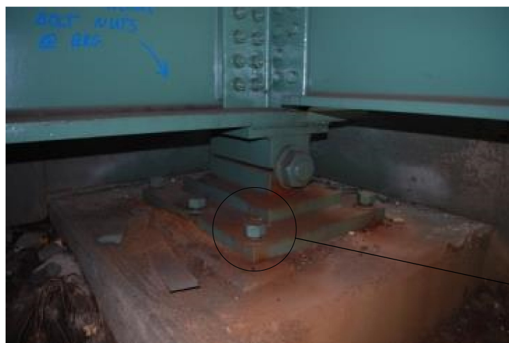
BRIDGE 10S EAST ABUTMENT BEARING ANCHOR BOLTS
