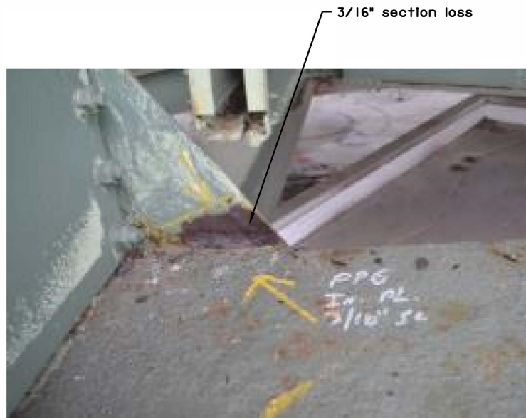
PANEL POINT 6, WEST TRUSS INTERIOR GUSSET PLATE LOOKING EAST
