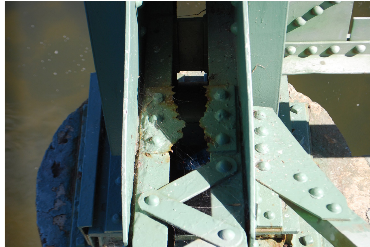
MEMBER L24, PIER 15 BATTEN PLATE IN WEST TRUSS (TYPICAL PHOTO)
