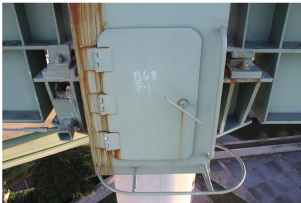
BRIDGE 68 PIER 1 - Hinge Repair
