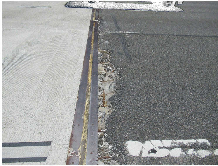
BRIDGE 8S - SOUTH ABUTMENT APPROACH SLAB
