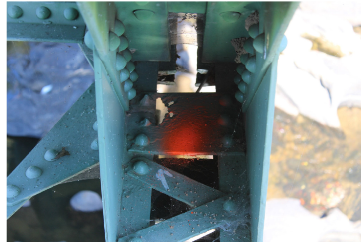
MEMBER L44, SPAN 12 BATTEN PLATE IN EAST TRUSS (TYPICAL PHOTO)
