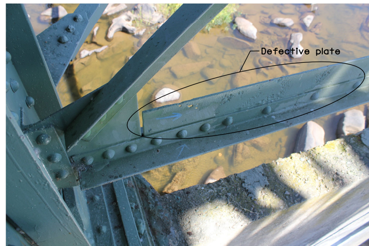
UNIT 11 LATERAL BRACING ANGLE IN WEST TRUSS
