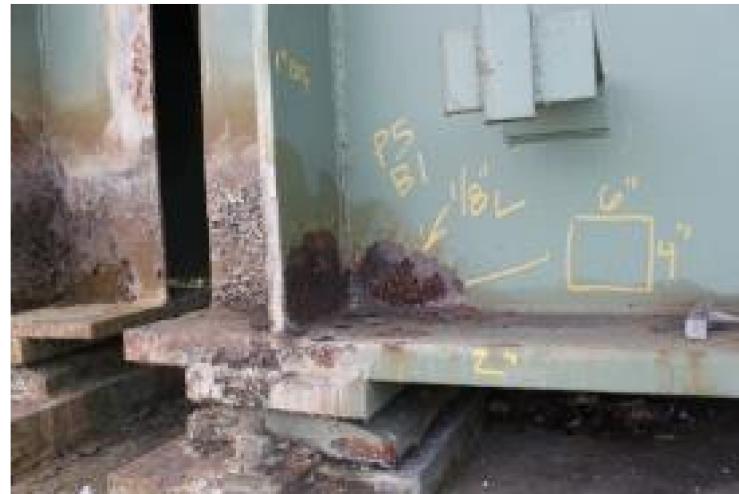
BRIDGE 5, PIER 5 STRINGER S33
