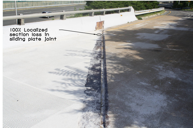
BRIDGE 17, NORTH ABUTMENT S-FLOYD
