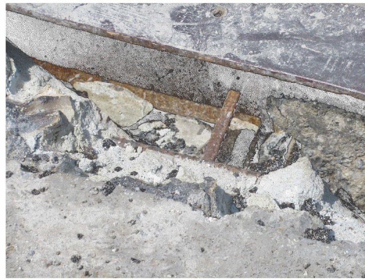
BRIDGE 8S SOUTH ABUTMENT APPROACH SLAB
