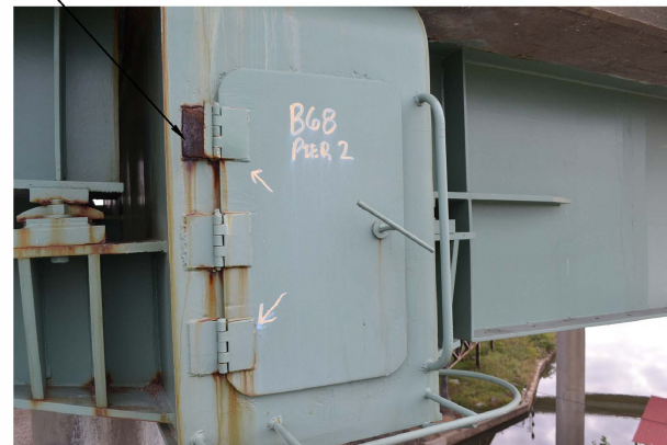
BRIDGE 68 PIER 2 - Hinge Repair
