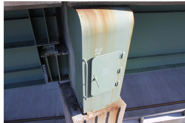
BRIDGE 66 PIER 16 - Hinge Repair
