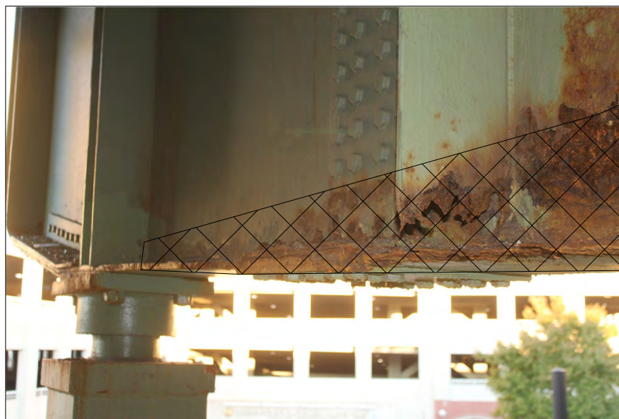
BRIDGE 67, PIER 12W FLOORBEAM 16 LOOKING NORTHWEST
