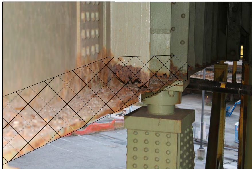
BRIDGE 67, PIER 12W FLOORBEAM 16 LOOKING EAST
