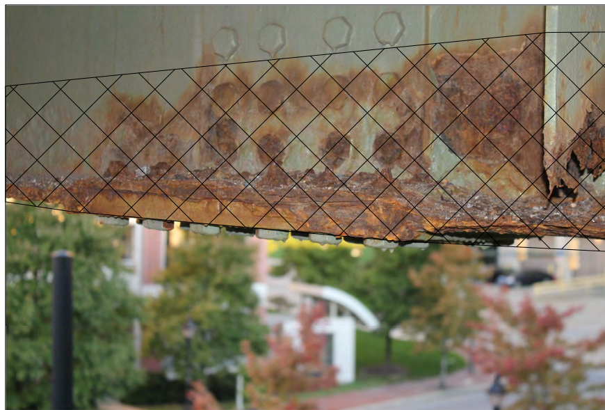
BRIDGE 67, PIER 12W FLOORBEAM 16 LOOKING NORTH
