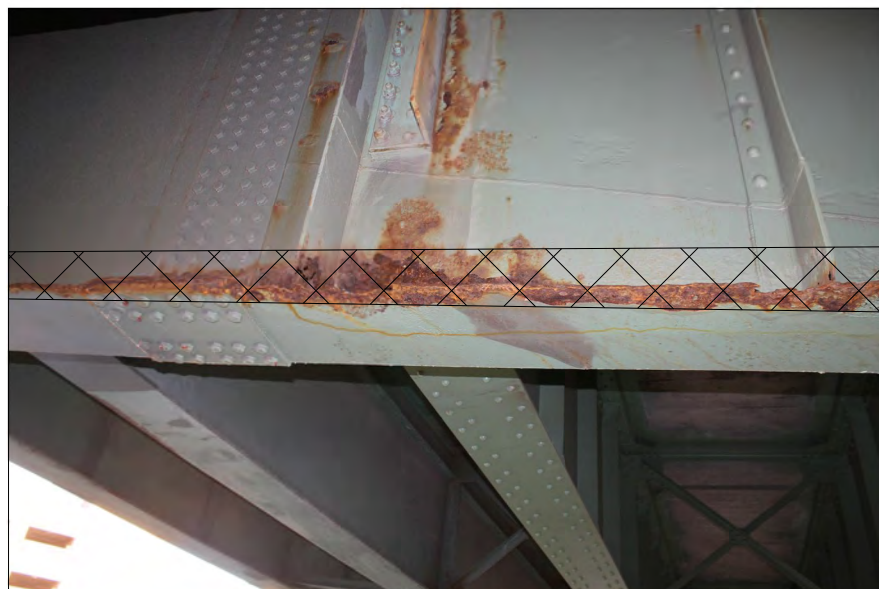
BRIDGE 67, PIER 12W FLOORBEAM 16 LOOKING NORTH
